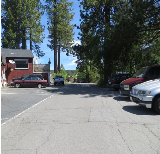
Mackinaw Road is a low volume street that provides an opportunity to have a shared environment between vehicles, pedestrians and bicyclists.
