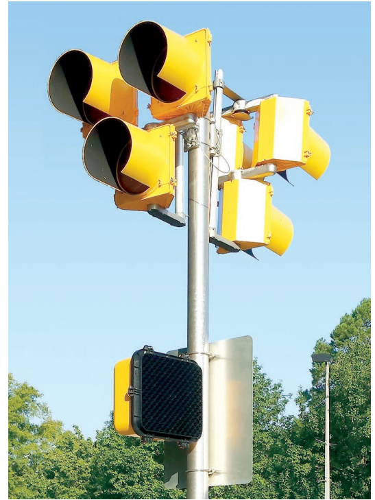
Example of a pole mounted PHB.
