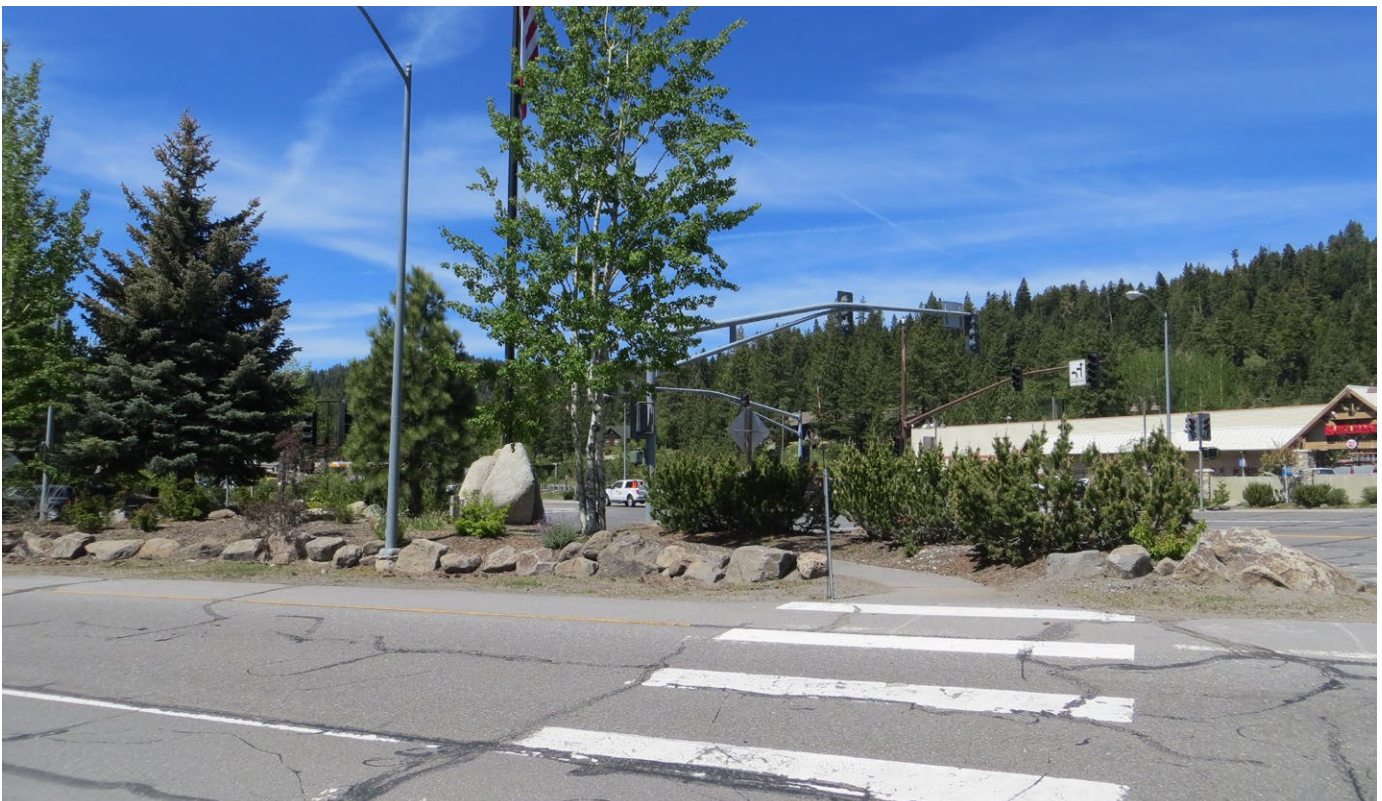
Most of the marked pedestrian crossings use high visibility style crosswalk pavement markings which enhance safety at the crossing location.
